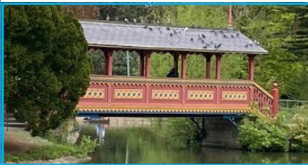
The "Swiss" Bridge
